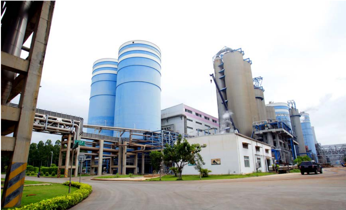
The area including the pulp making mill is seen. The left building is bleached pulp tower and right one is bleaching stage at the APP's (Asia Pulp and Paper) Hainan pulp and paper mill in Yangpu, China. The complex includes the biggest pulp mill in China. Mike De Sisti, Milwaukee Journal Sentinel
